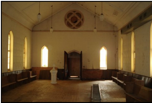
The inside of the church: the floor must be removed and foundational work done. The church needs heat, air conditioning, water, and electricity.
